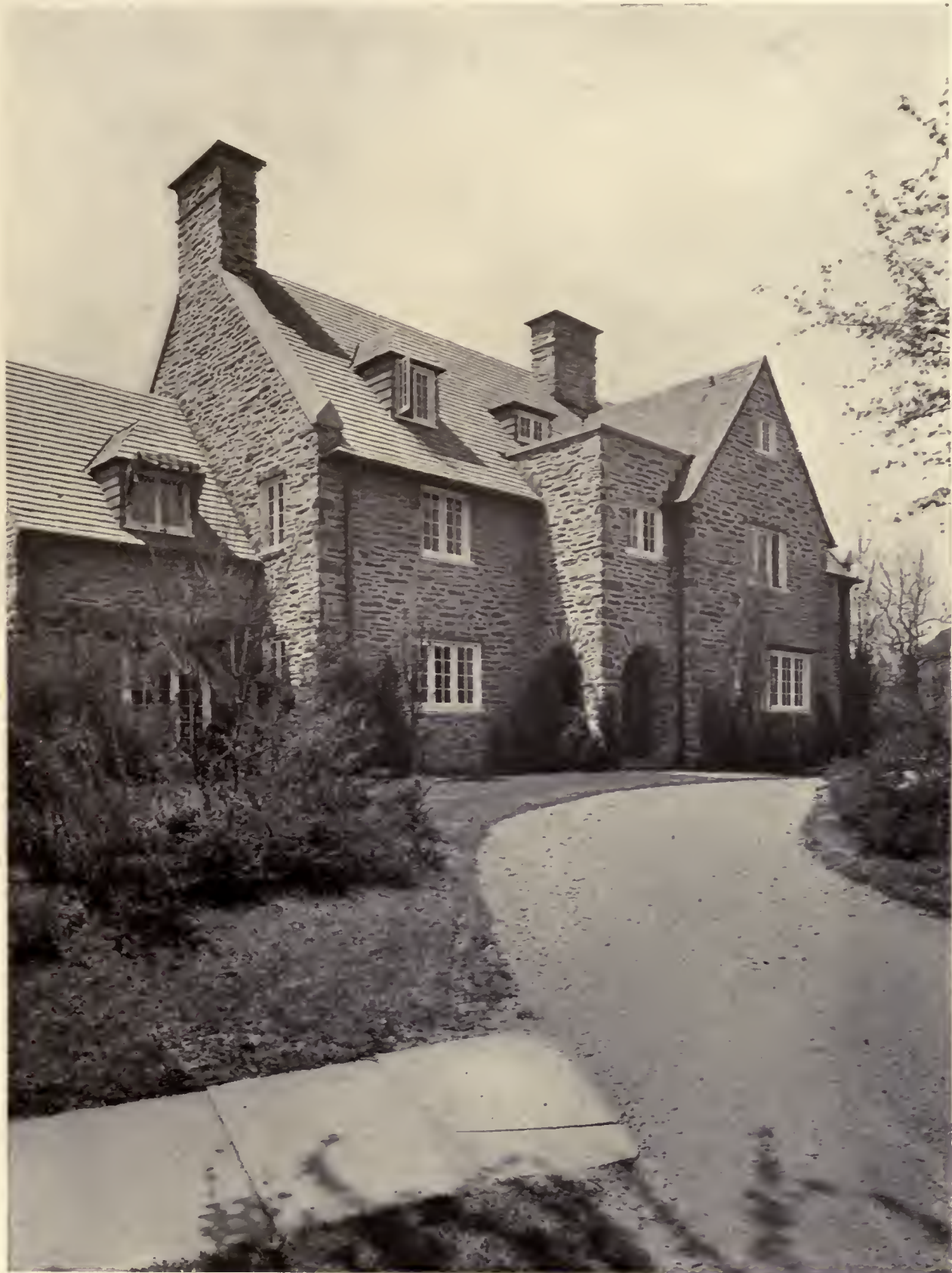
HOUSE OF MR. NORMAN ELLISON, CHESTNUT HILL, PA. ROBERT R. MCGOODWIN, ARCHITECT
